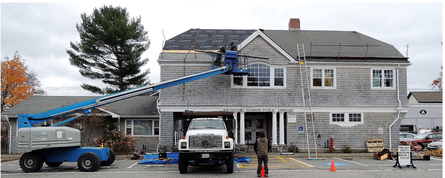
Ground crew monitoring the Village Green Entrance while replacing shingles
