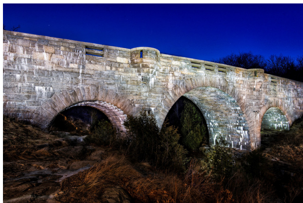
Duck Brook Carriage Road bridge, 2012 Photographer — Howie Motenko
